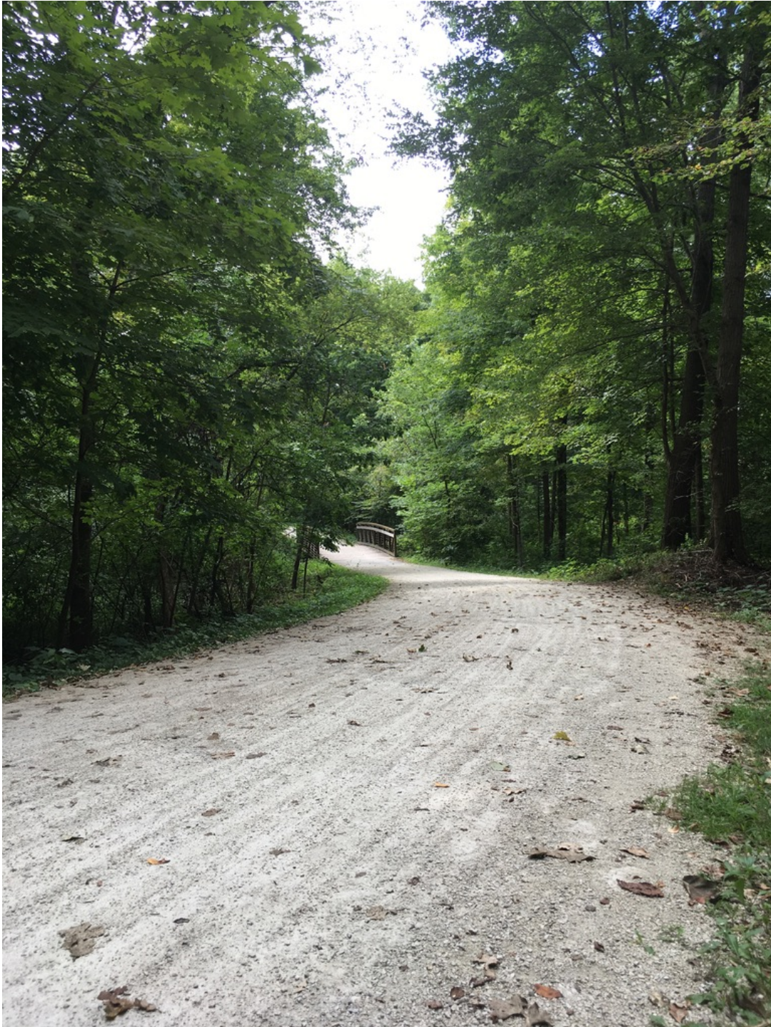
Bridge across Big Bremme Creek and the trail leading to the clearing Photo by Donna Kubik
