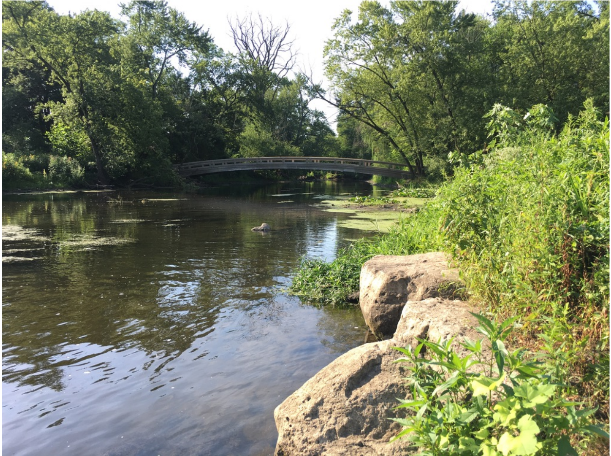
Bridge crossing over the West Branch of the DuPage River Photo by Donna Kubik
